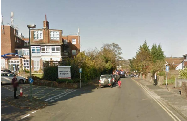
Figure 4. Looking north towards the A25 (Seal Road) on Hospital Road.
